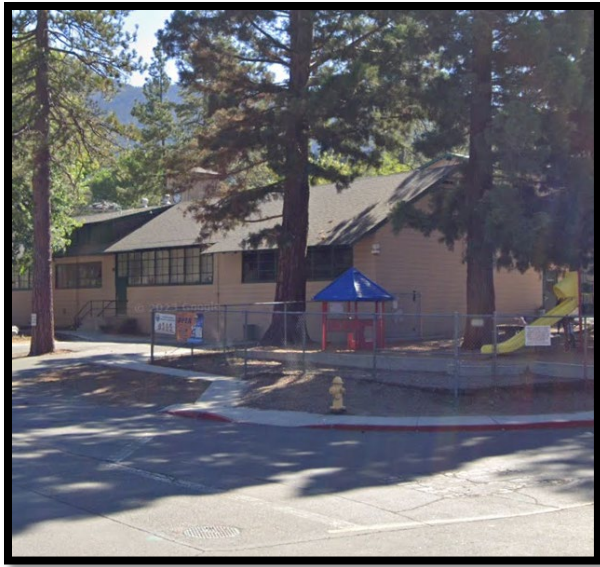
Figure 4 Idyllwild School curb ramp photo
